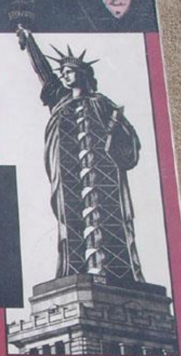
The interior framework designed by Eiffel
